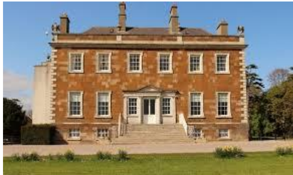
NEWBRIDGE HOUSE & FARM DONABATE, CO. DUBLIN
